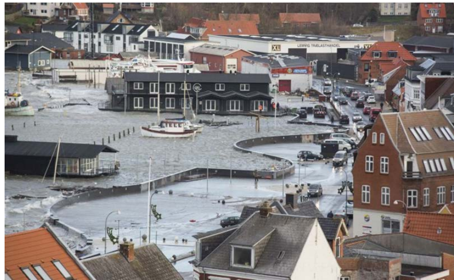
Storm surge wall in town of Lemvig, Denmark
